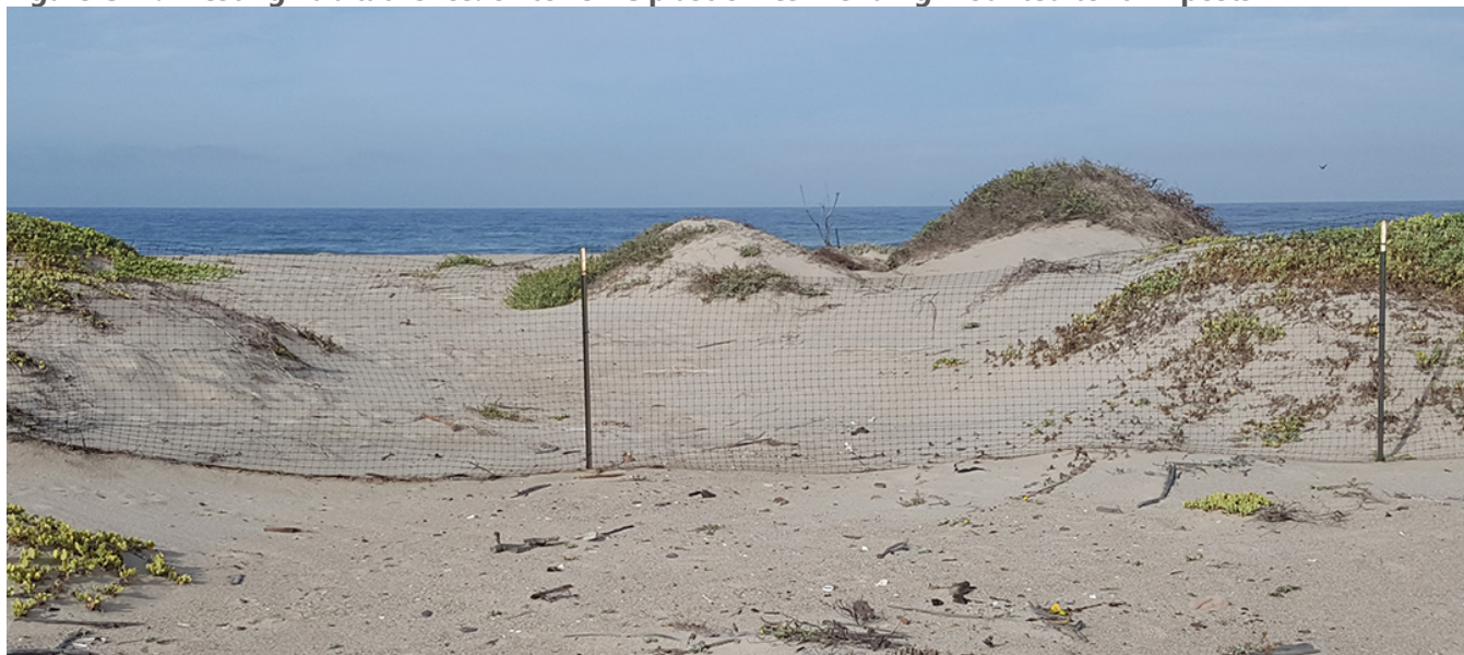
Figure C- 1. Nesting habitat fence: cintoflex-C plastic mesh fencing mounted to 6' T-posts
